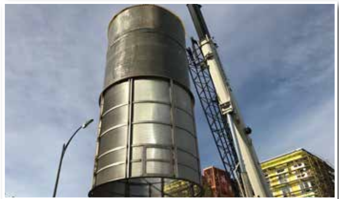
CDS standalone system removes trash and sediment.
