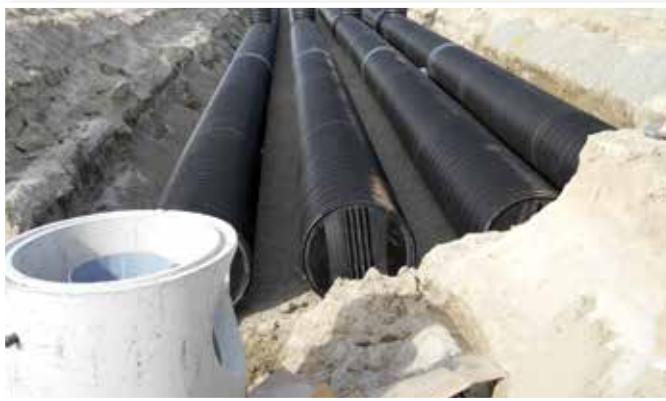
CDS pretreats a rainwater harvesting cistern.
